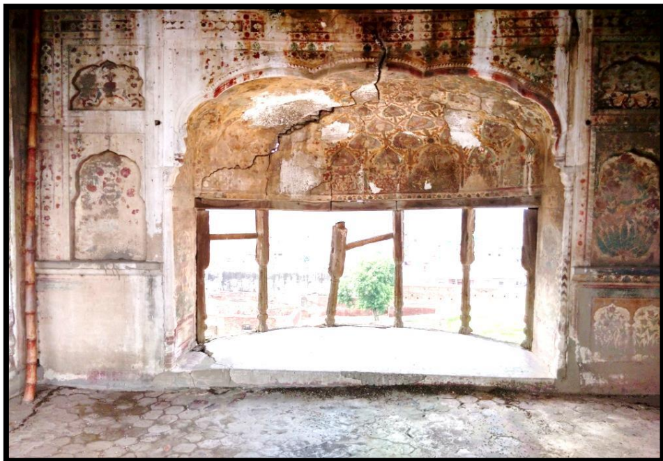
Inside haveli Cracks and damaged plaster
